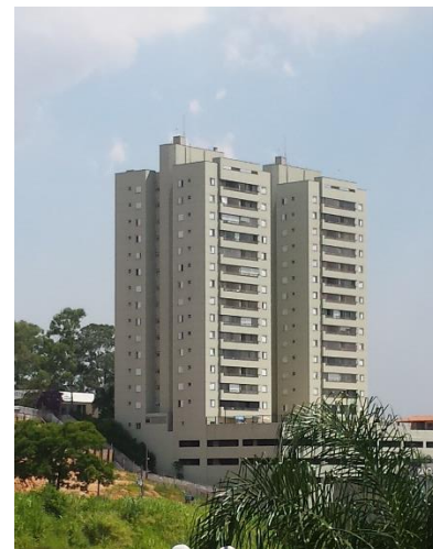
Fig. 1. Identical buildings (P2 on the left, P1 on the right), both have the same LPS installed.
