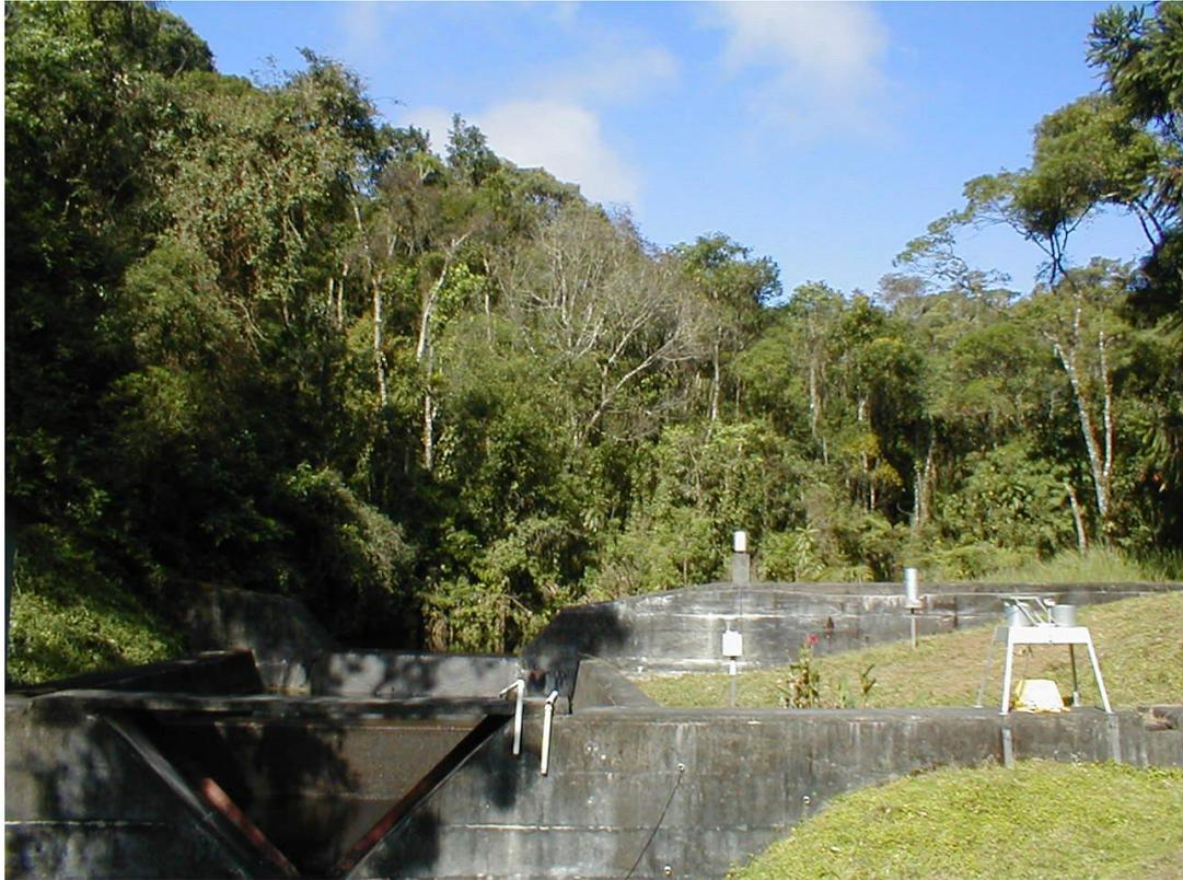
Figure 3b. Weir installed at the CUNHA stream B watershed (Forti, 2000).
