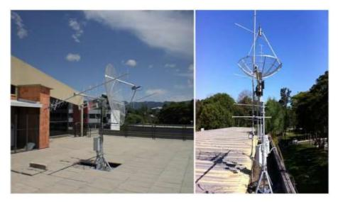
Figure 2: The NANOSATC-BR's Ground Station Network (GS) is already installed and in operations: on left - GS(INPE-CRS) at CRS/INPE-MCTIC, in Santa Maria, RS, and *on right* - GS(INPE-ITA) at ITA/DCTA-MD, in São José dos Campos, SP, in Brazil.
